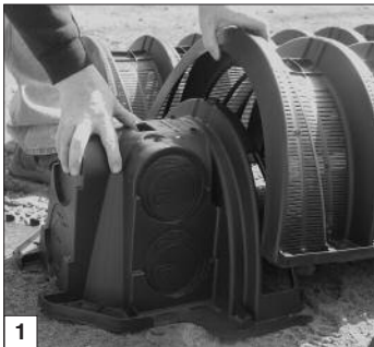
Slide end cap under chamber.
