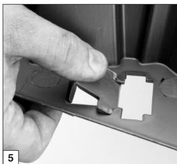
5 Activate StraightLock Tabs.
