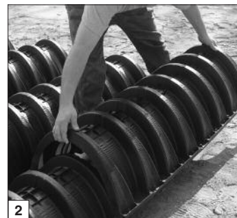
Connect the chambers.
