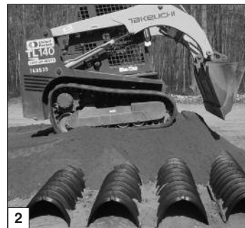
Build ramp of soil.
